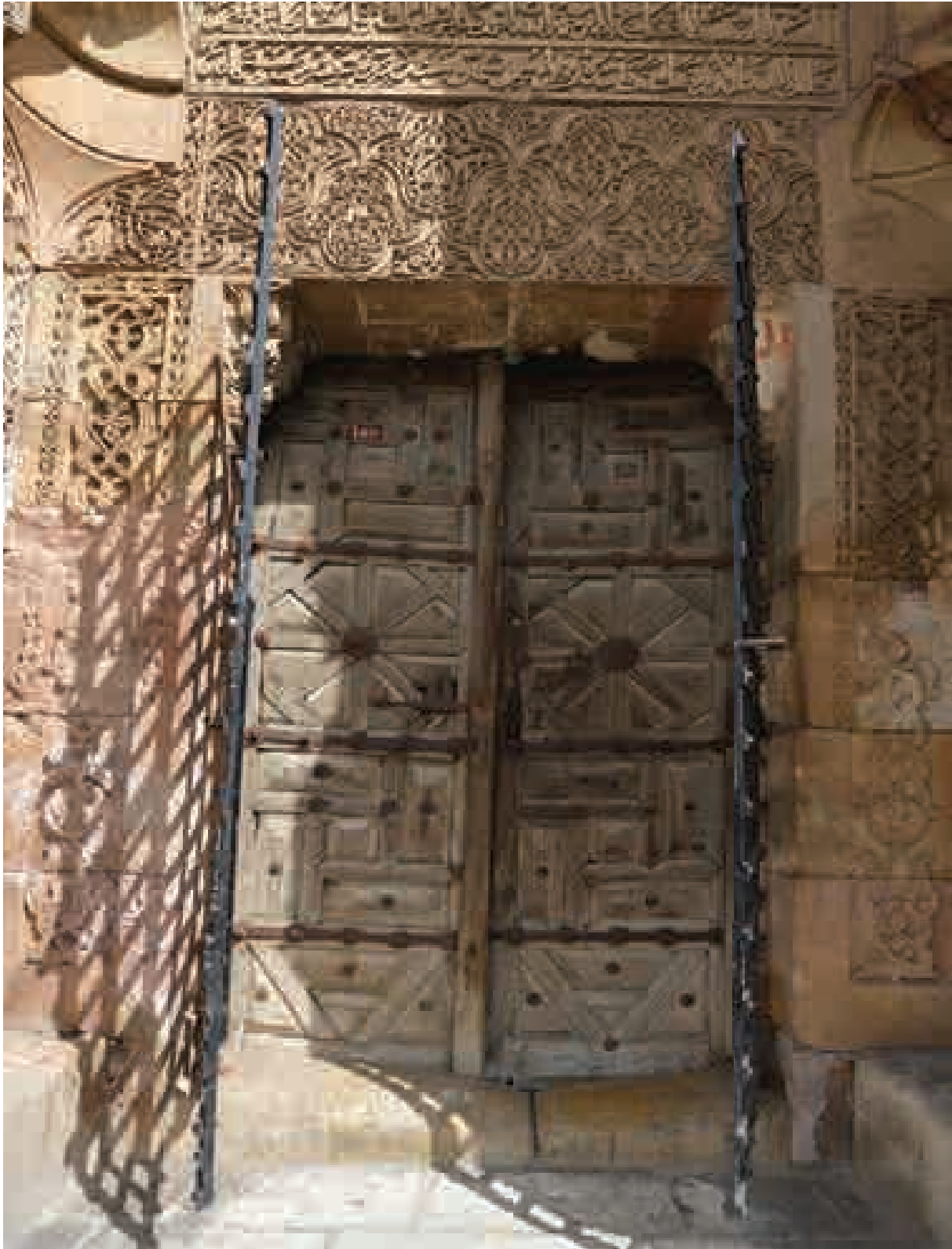
Carved stone decorations on the portal of the hospital
