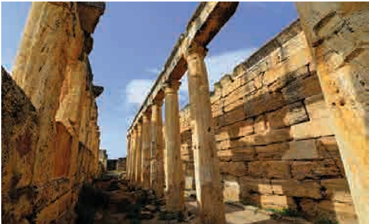
Toilet / the Latrina building
