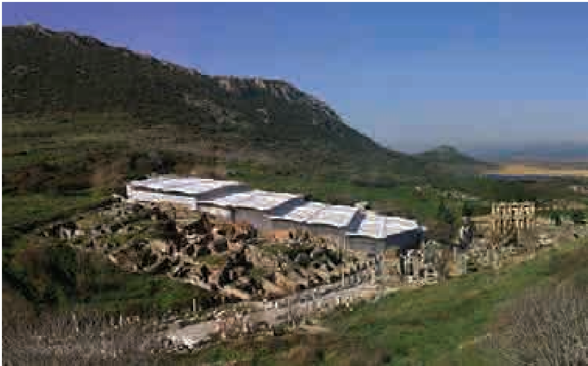
Terrace Slope House 2 protective roof in 2015 (Austrian Archaeological Institute, Niki Gail)
