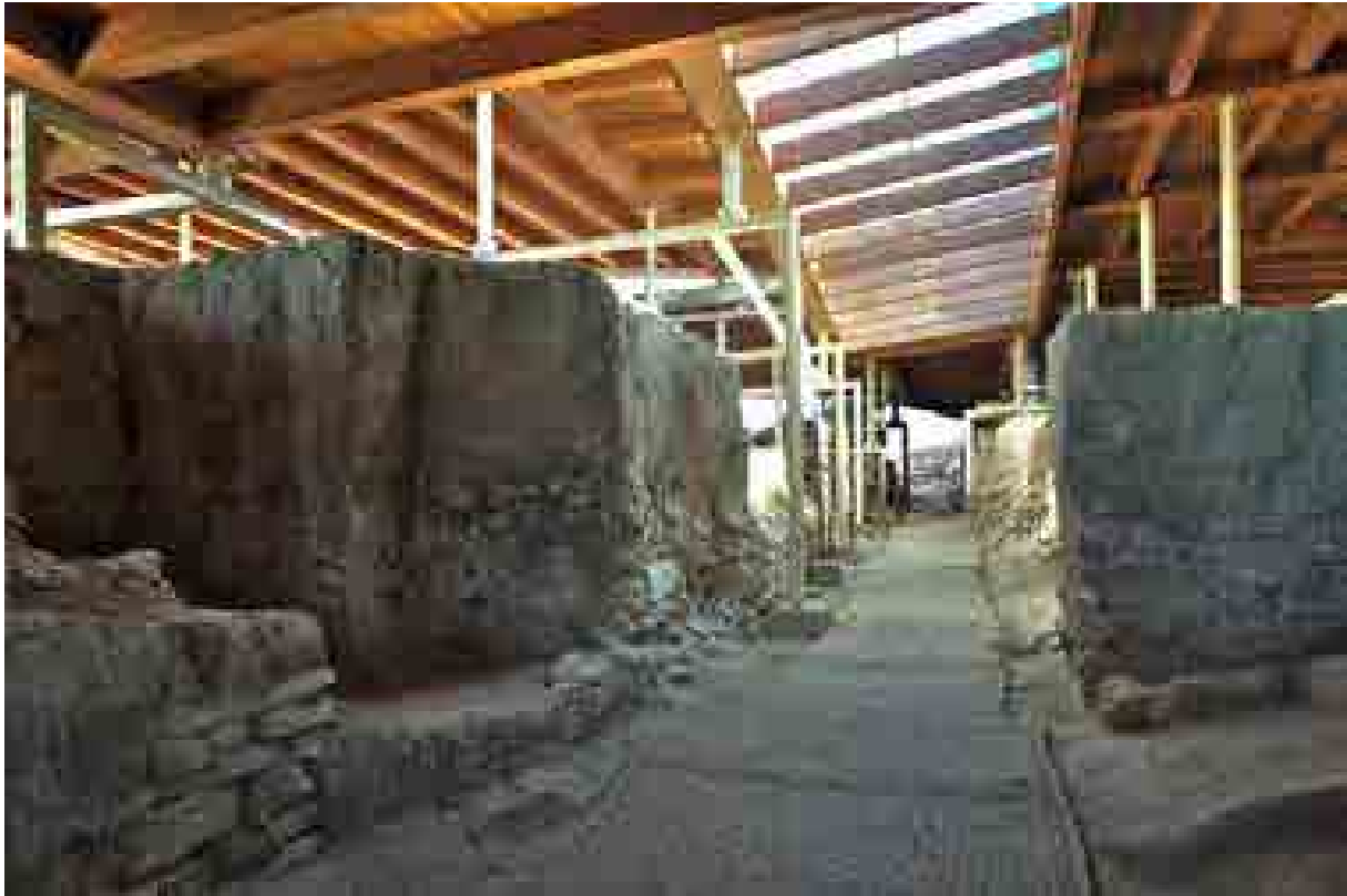
The permanent roofing system covering and protecting the fourth millennium Palace, view of gate and corridor from inside (MAIAO)
