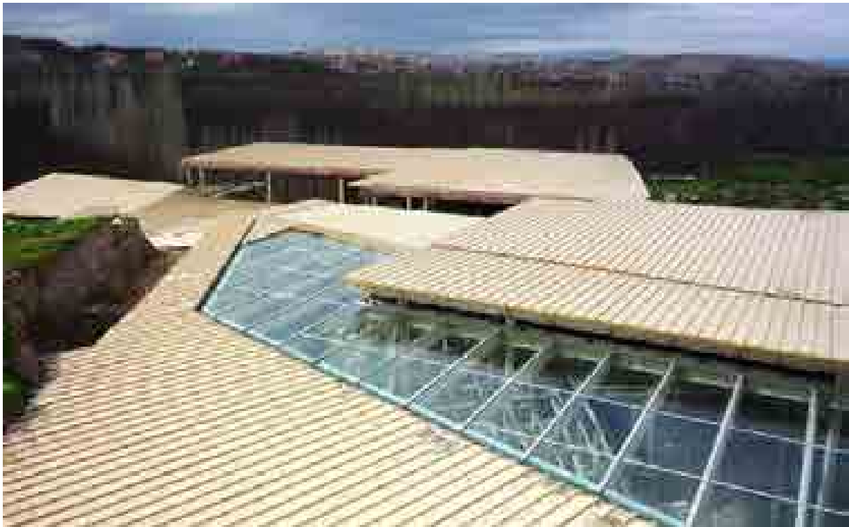
View of the roof from the top of the mound (MAIAO)
